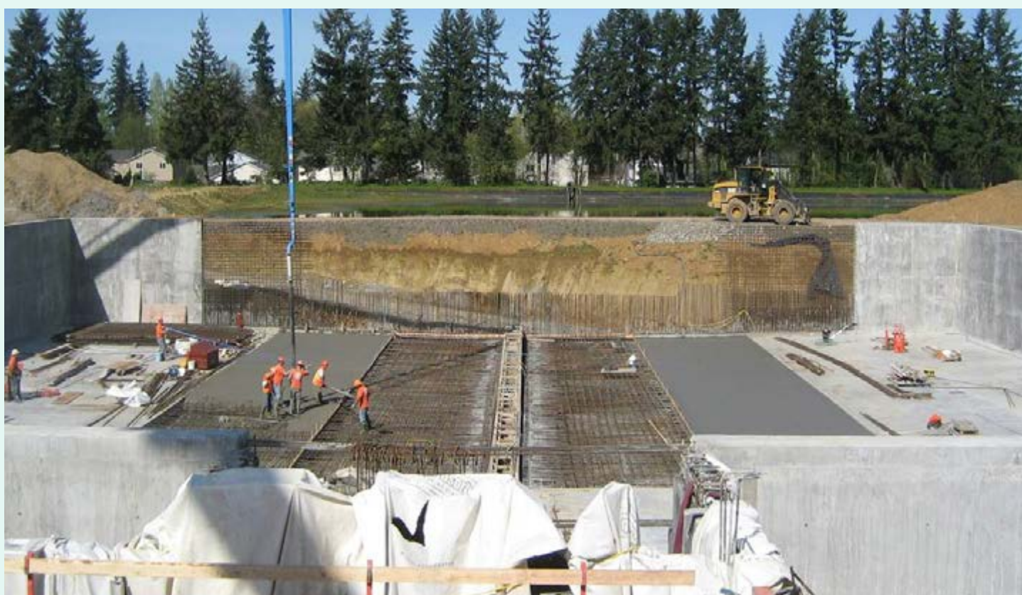
Equalization basin for Battle Ground forcemain (2015)
