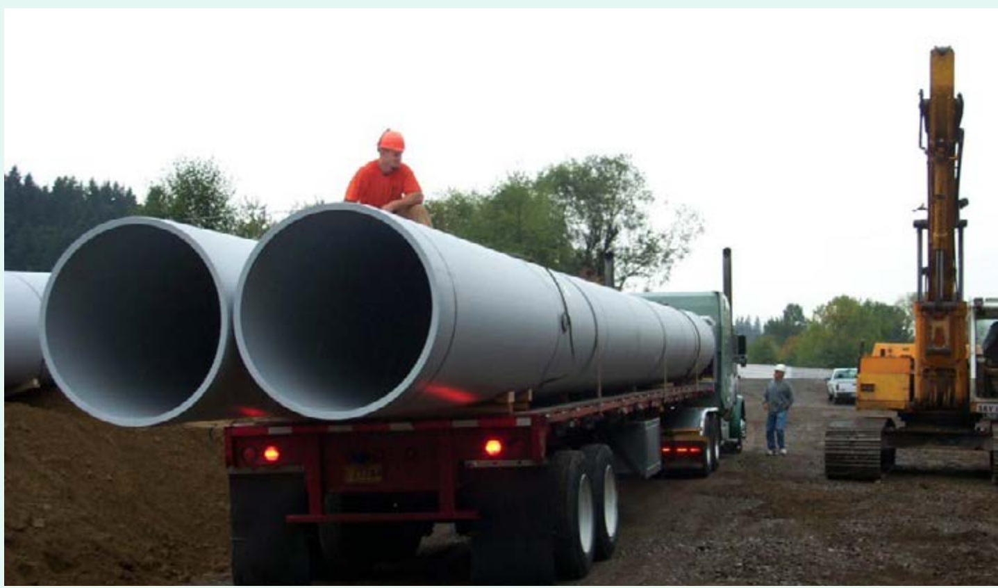
Installation of Kline Interceptor (2004–2007)
