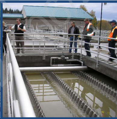
Existing Primary Clarifier
