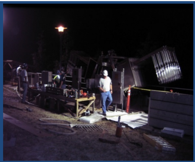
Existing UV System Expansion During Phase 4
