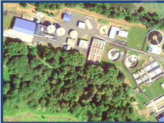
Salmon Creek Treatment Plant Aerial
