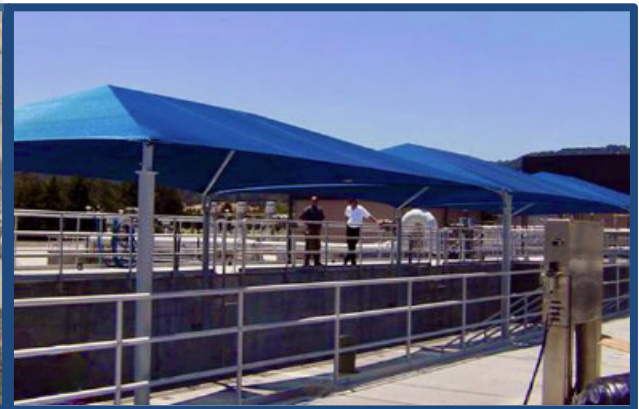
Example Solar Shading Equipment
