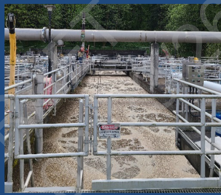
Existing Aeration Basins 5 & 6
