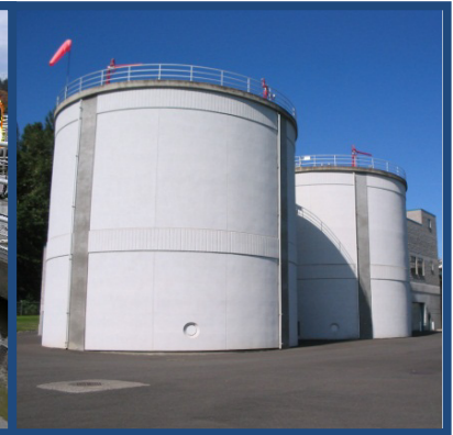
Existing Anaerobic Digester
