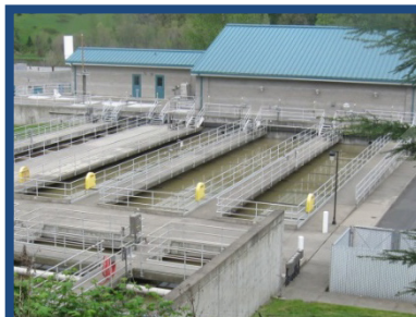
Existing Primary Clarifiers
