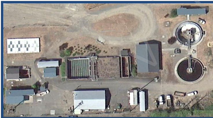
Ridgefield Treatment Plant Site
