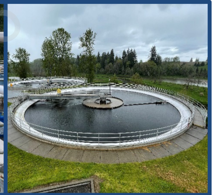
Existing Secondary Clarifiers 3 & 4
