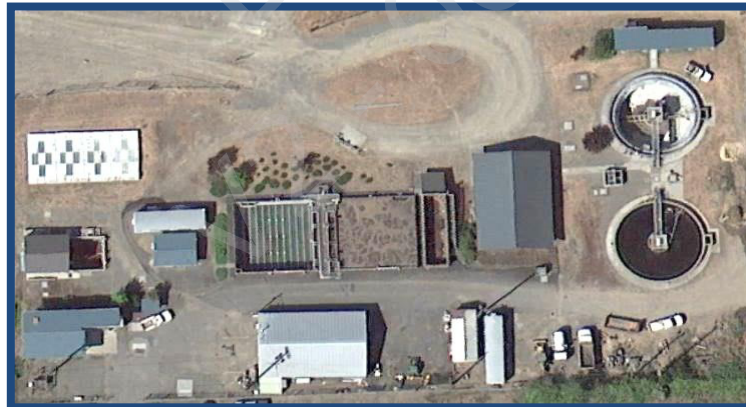
Ridgefield Treatment Plant Site
