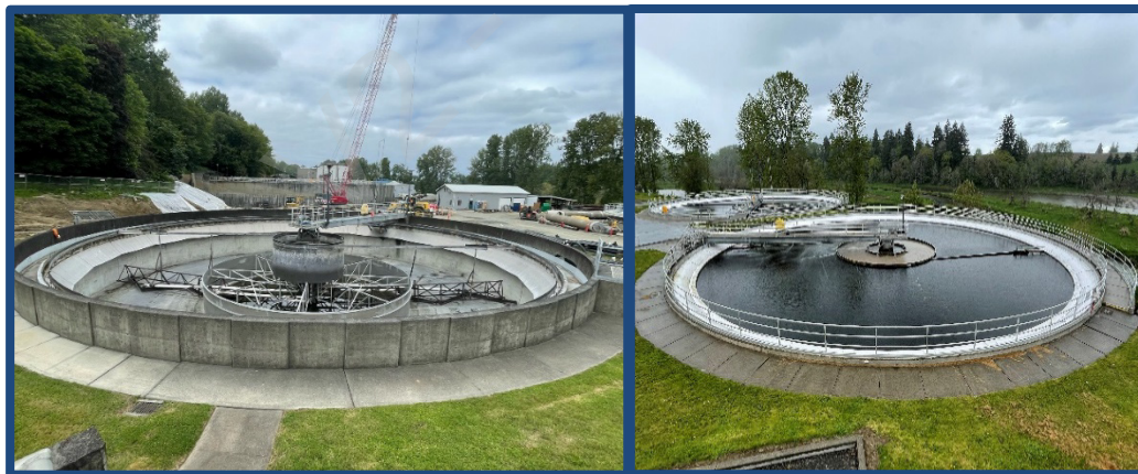
Existing Secondary Clarifier 1
