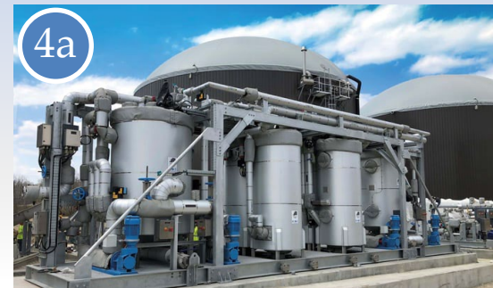
Thermal Hydrolysis Process (THP) “Pressure cooker”
