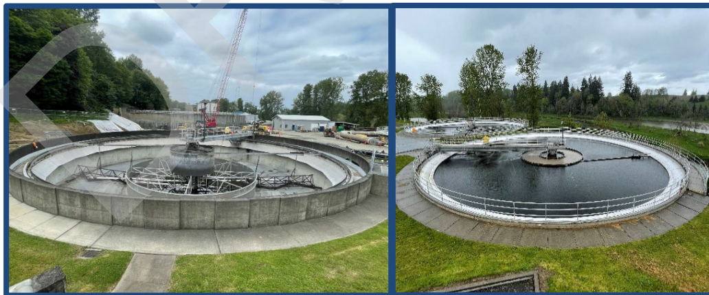
Existing Secondary Clarifier 1
