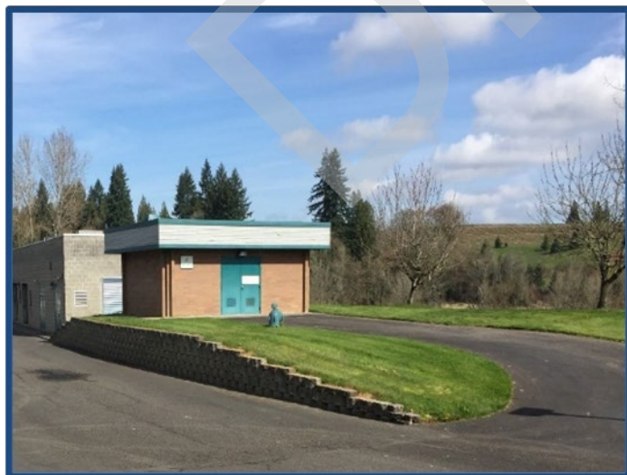
Existing SCTP Well House for Potable Water Supply
