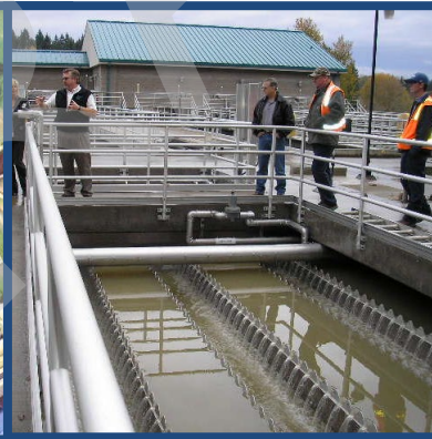
Existing Primary Clarifier
