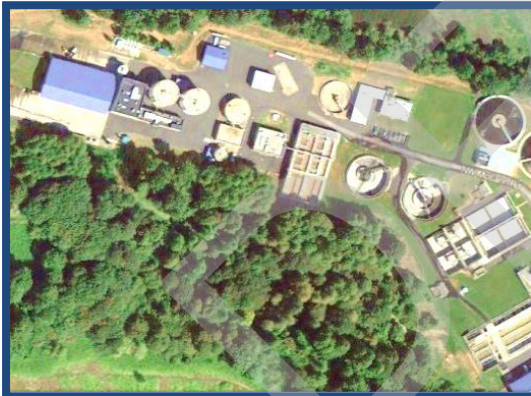
Salmon Creek Treatment Plant Aerial
