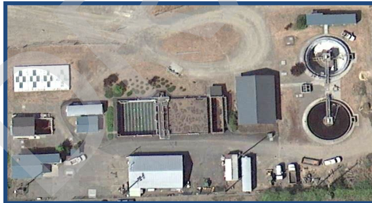
Ridgefield Treatment Plant Site
