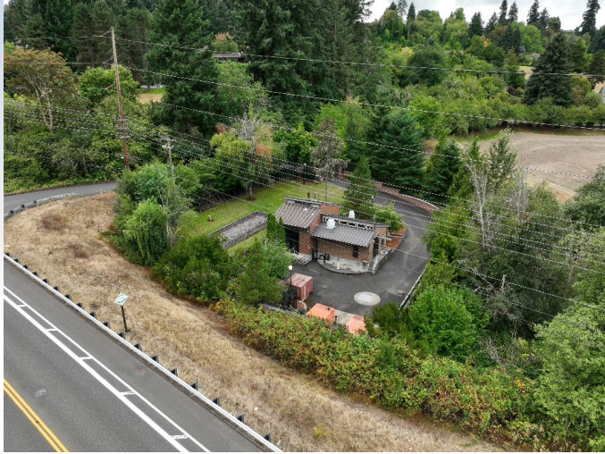
36 th Avenue Pump Station
