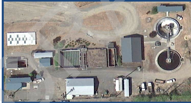
Ridgefield Treatment Plant Site
