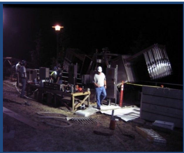
Existing UV System Expansion During Phase 4
