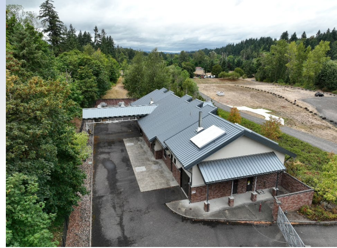
117 th Street Pump Station
