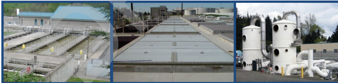
Existing Primary Clarifiers
