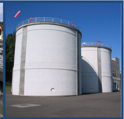
Existing Anaerobic Digester
