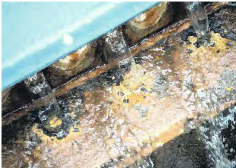
Clean water falls over a weir in a secondary clarifier tank at the plant.
