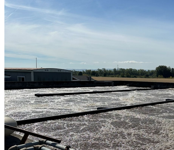
RTP's South Aeration Basin with flow baffling installed.
