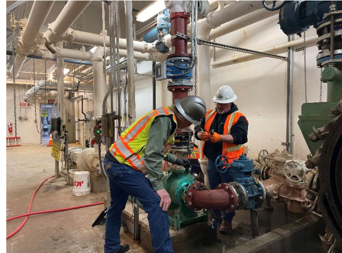
Representatives from Pumptech and Vaughn assess the digester recirculation pumps.
