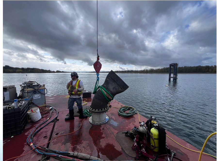
Diffuser and new riser
