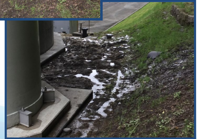
Drainage Issues behind Sludge Blend Tank
