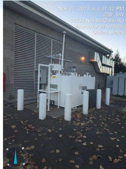
New Diesel Tank
