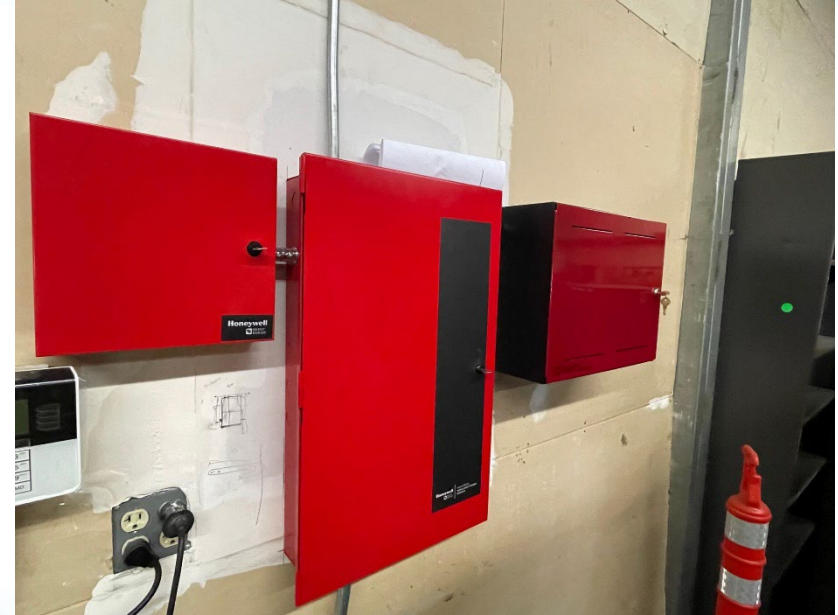
New Fire Alarm Panel
