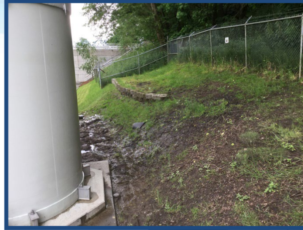
Drainage Issues behind Sludge Blend Tank
