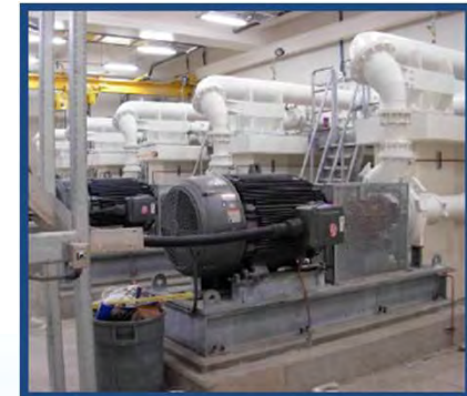
117 th Street Pump Station & existing pump assembly
