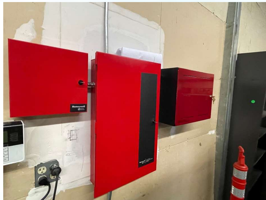
New Fire Alarm Panel
