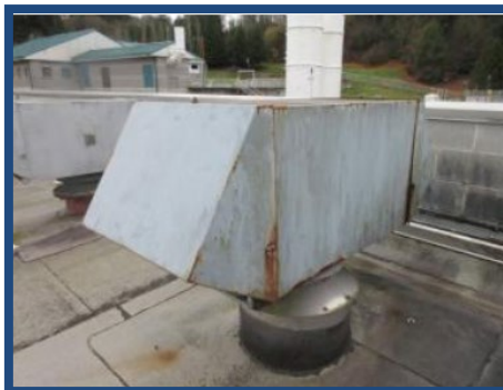
SCTP Corroded Supply Fan
