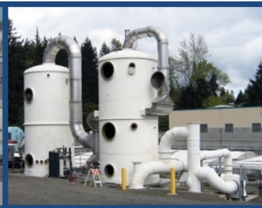
Bio Trickling Filter Tower
