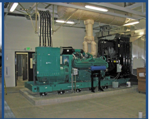
Existing Engine Generator
