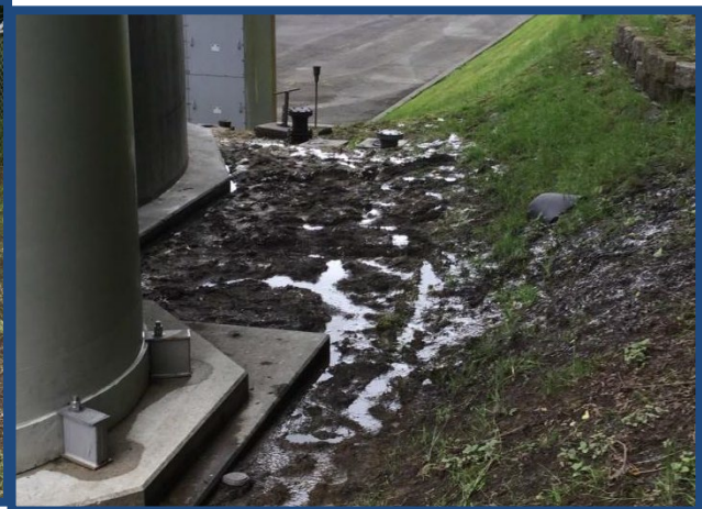
Saturated Ground At Foundation
