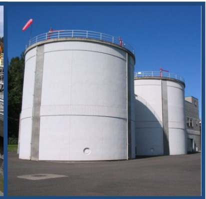
Existing Anaerobic Digester
