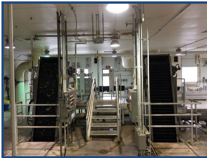
Existing Influent Screens Rebuilt in 2017
