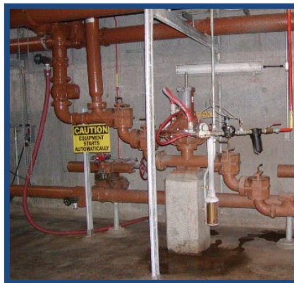
Existing Diaphragm Style Pump
