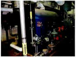
5.c <u>Fulton Pulse Boiler</u>. This boiler is a Fulton Pulse Combustion model PHW-750, fired on natural gas. The boiler is equipped with Leeson burners rated at 0.75 MMBtu/hr and is used to heat the administration building. This boiler was installed in 1996.
