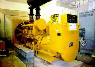
5.i Flow Augmentation Pump Engine #1. This diesel engine is used to power a wastewater pump used only during high peak flows. Specific engine information is listed below:
