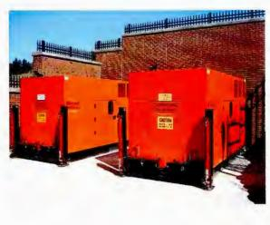
Flow Augmentation Pump Engine #2. This diesel engine is 5.j used to power a wastewater pump used only during high peak flows. Specific engine information is listed below:
