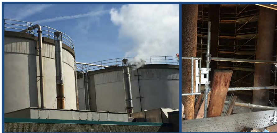
Digesters at Salmon Creek Treatment Plant
