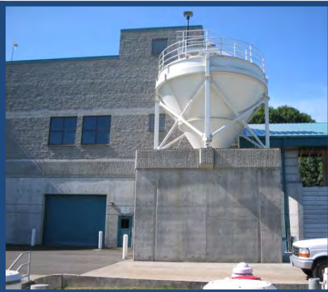
Sctp Solids Processing Center
