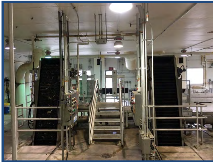
Existing Influent Screens Rebuilt in 2017
