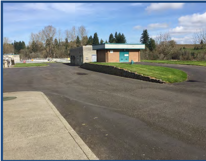
Paved Area Near the Headworks Building
