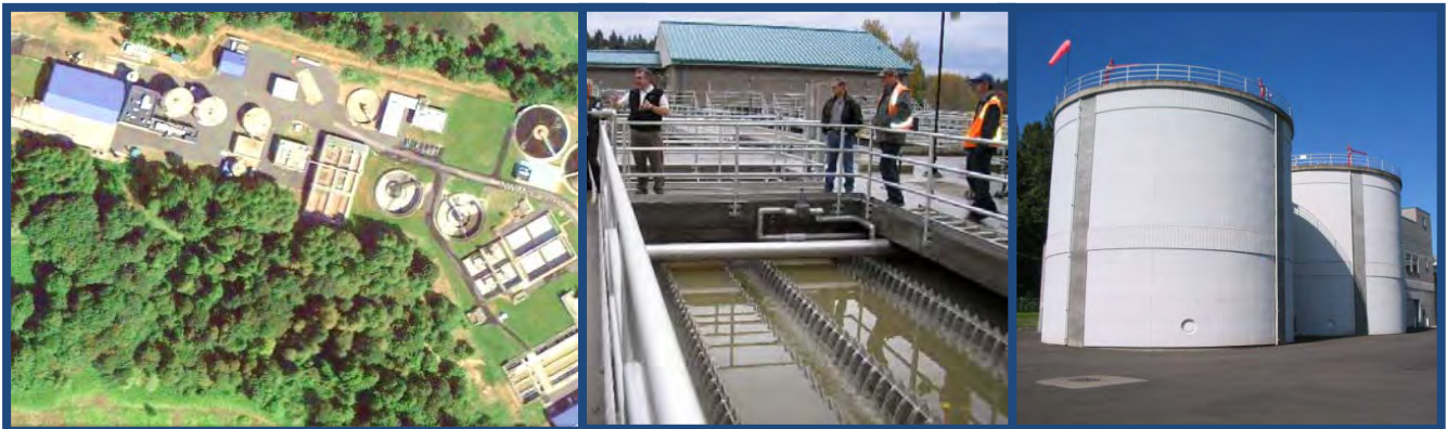
Salmon Creek Treatment Plant Aerial
