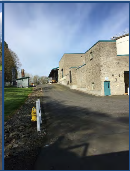
Paved Area Near the Solids Building
