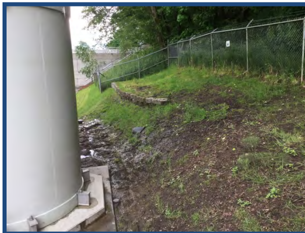
Slope South of Sludge Blend Tank
